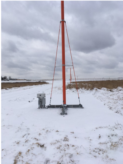
Completed light tower
