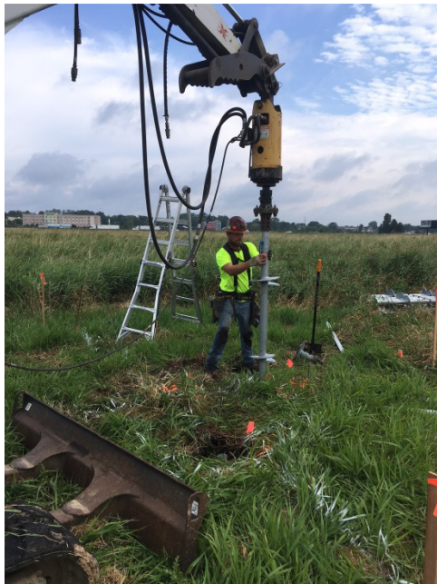
Helical pile for approach light tower
