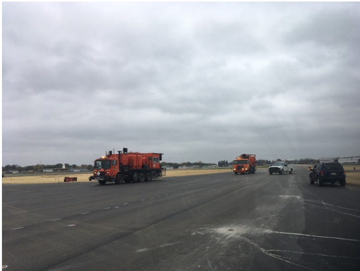
Runway Paint Marking
