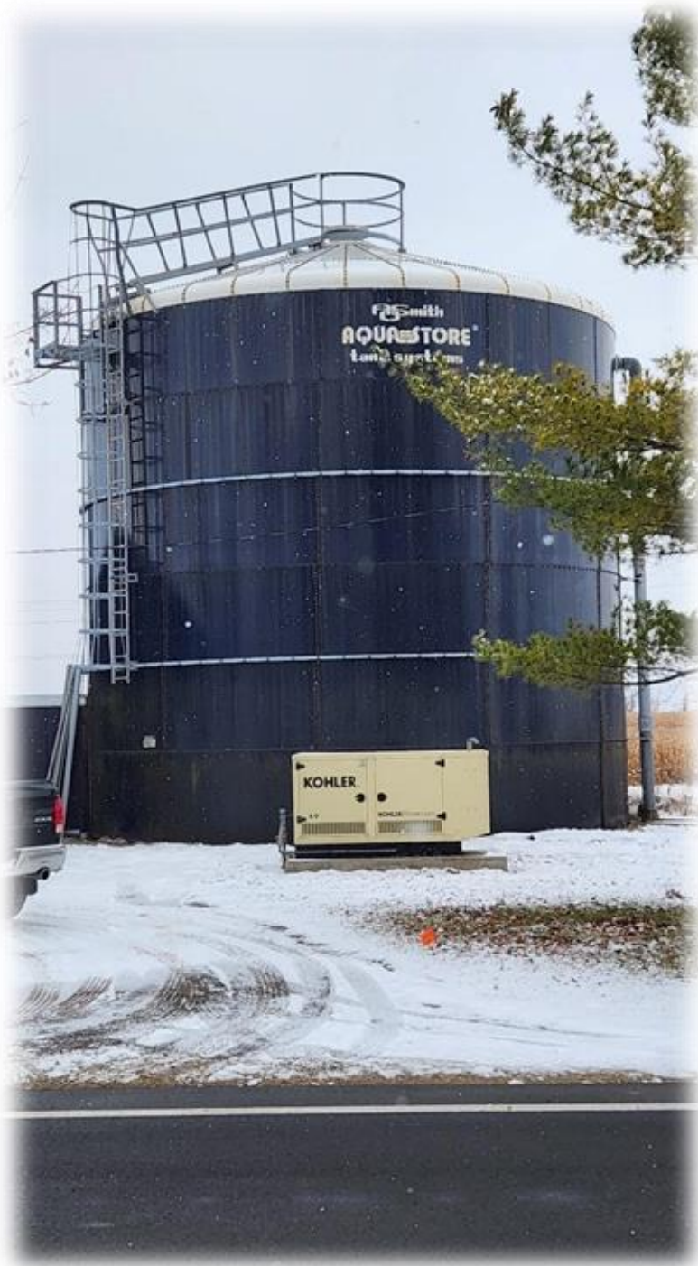
New Water Tower
