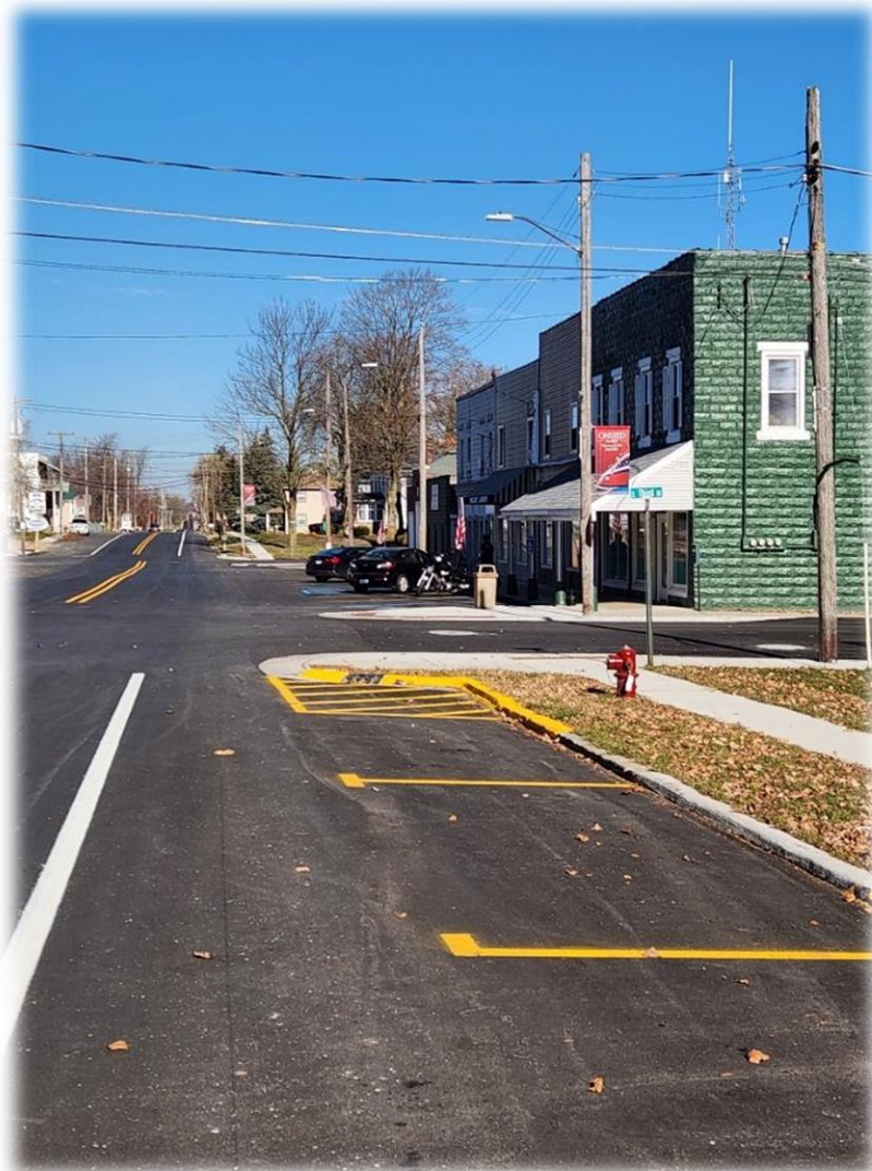
Street Paving Project, Downtown Onsted 2023
