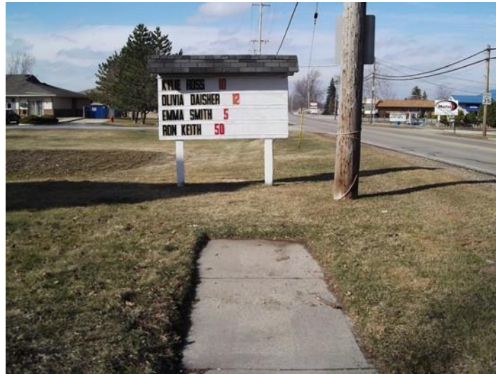
Sidewalk along west side of Main Street terminating just south of Wexford Manor
