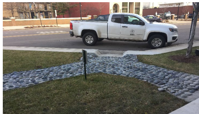
Figure 13-3 An Example of Storm Water Management in the City of Jackson
