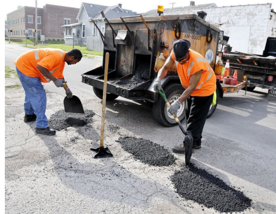
Figure 10-2 Filling Potholes
