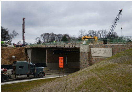
Figure 6-4 Cooper Street Bridge under Construction
