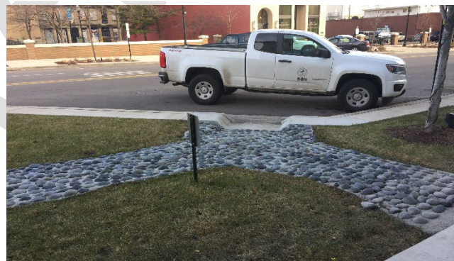
Figure 13-6 An Example of Storm Water Management in the City of Jackson
