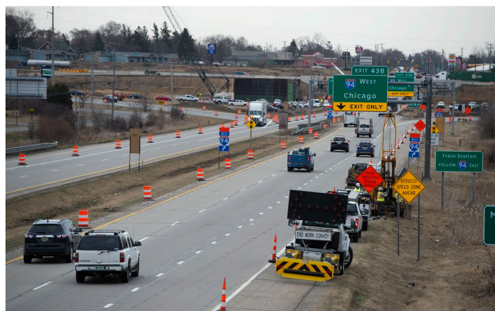
Figure 10-3 Construction on US-127
