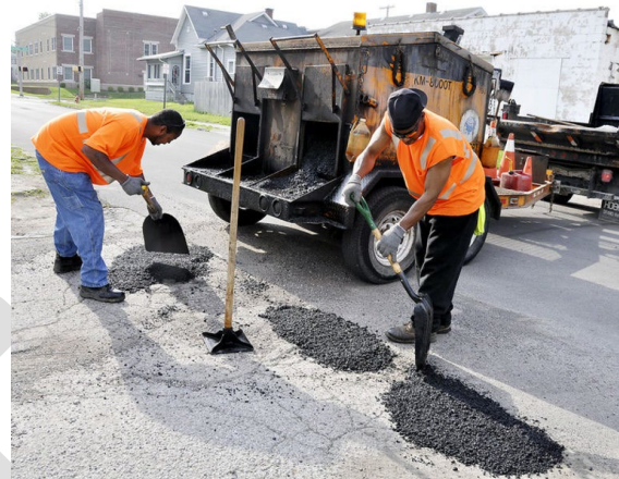
Figure 10-2 Filling Potholes
