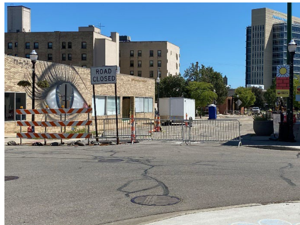
Figure 4-3 Cortland Street under Construction
