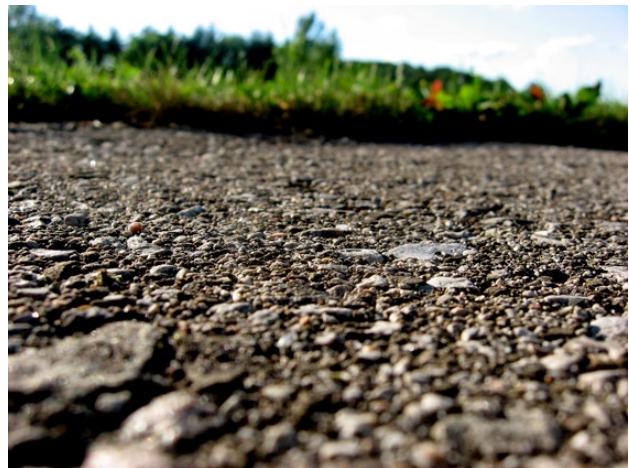
Figure 10-1 Weathered Asphalt Road
