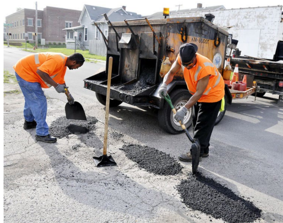
Figure 10-2 Filling Potholes
