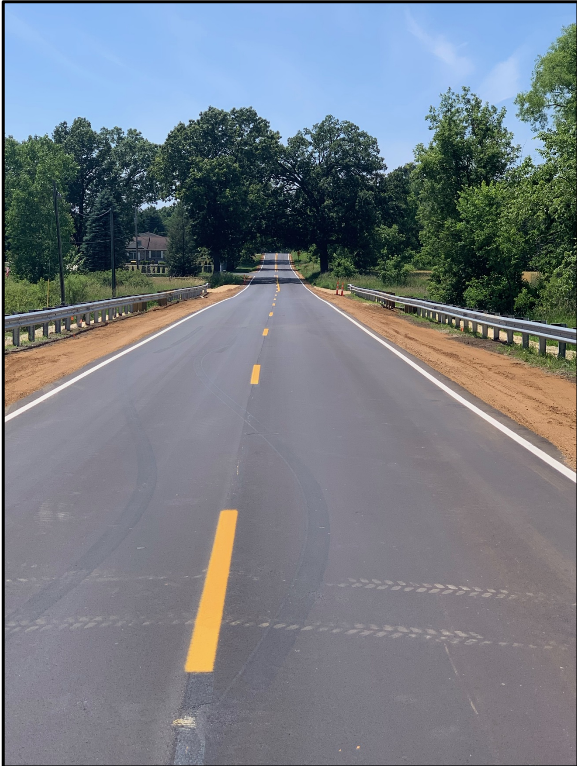
Territorial Road (Section of Upgraded Guardrail to Current Standards)
