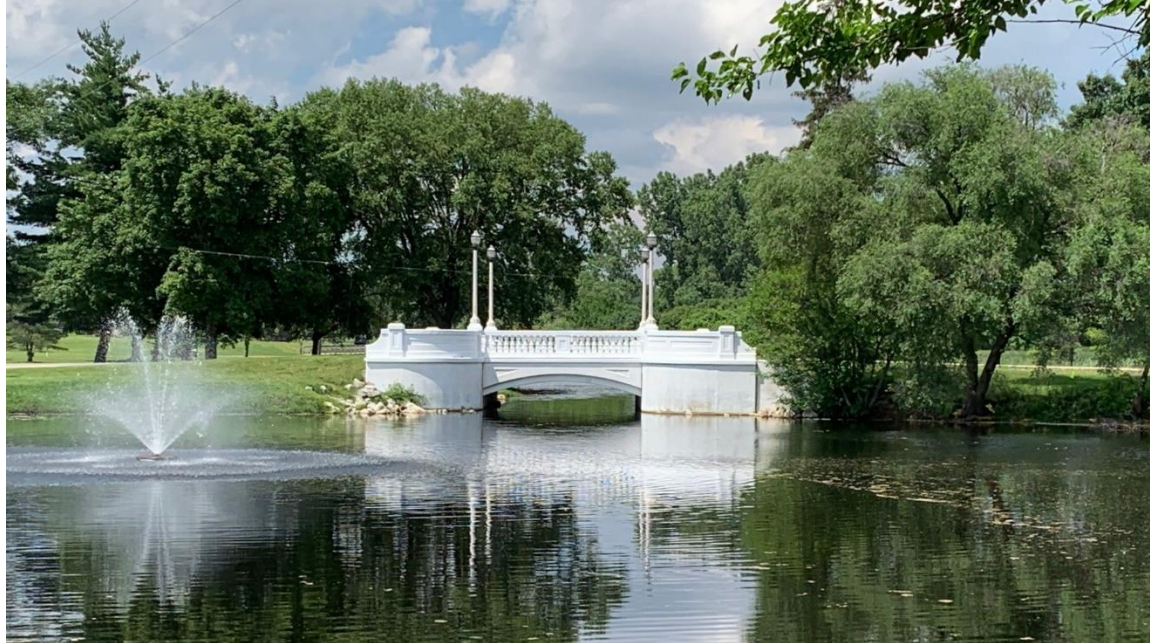
Denton Road Bridge | Sparks Foundation County Park
