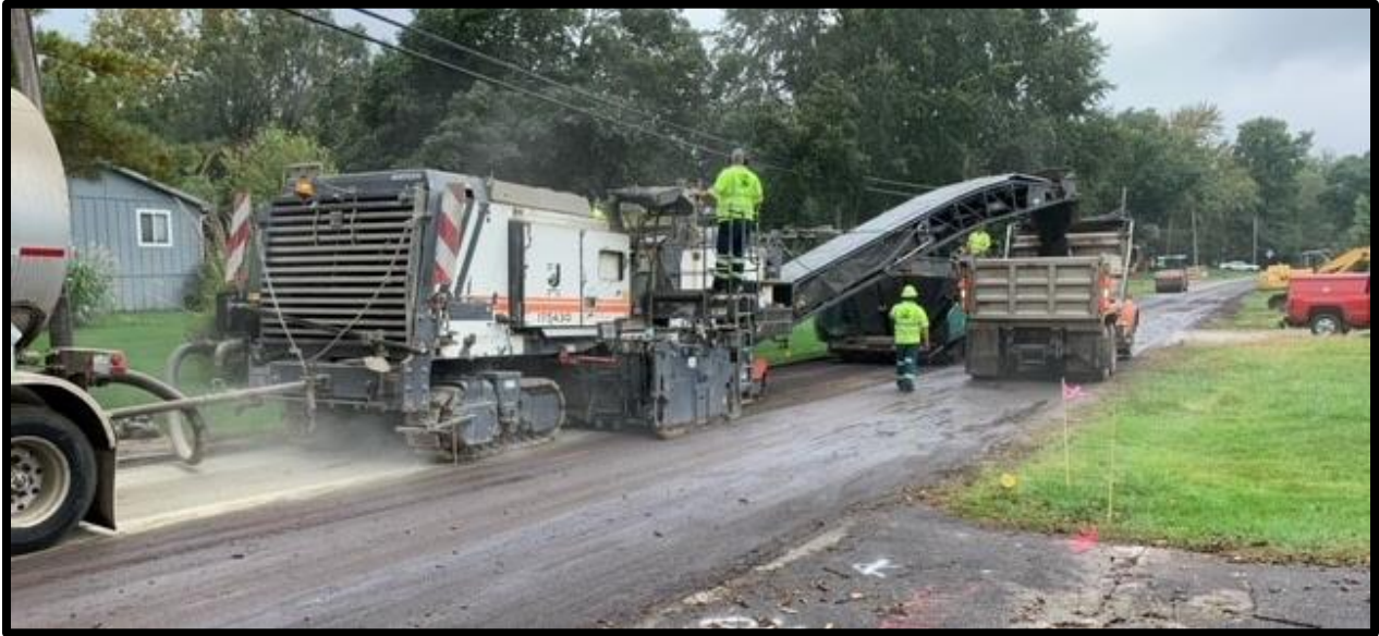
McCain Road – Cold-in-Place Recycling Operation
