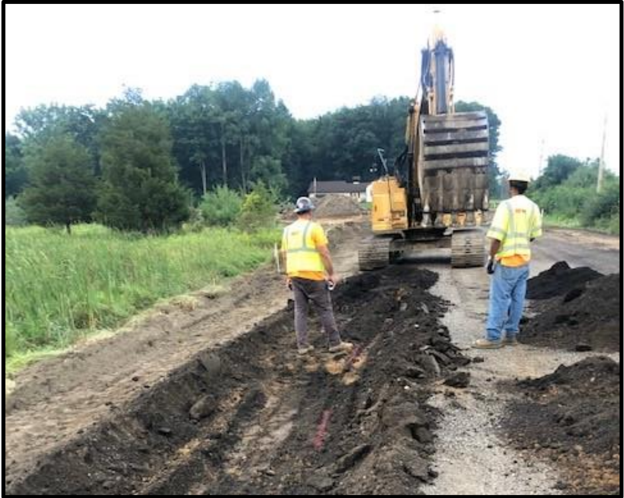
S. Jackson Road at Lindsey Road – Removing existing organic soil
