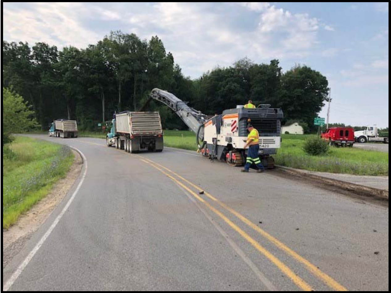
S. Jackson Road at Lindsey Road – JCDOT crews removing existing curve for future use
