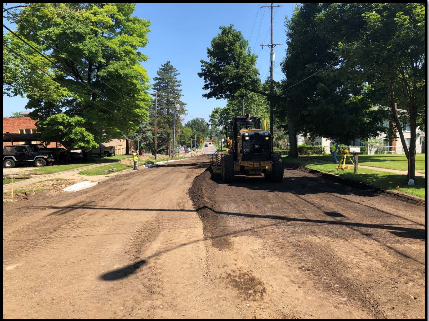
Village of Grass Lake, Union St. south of Michigan Ave – Grading the crushed material
