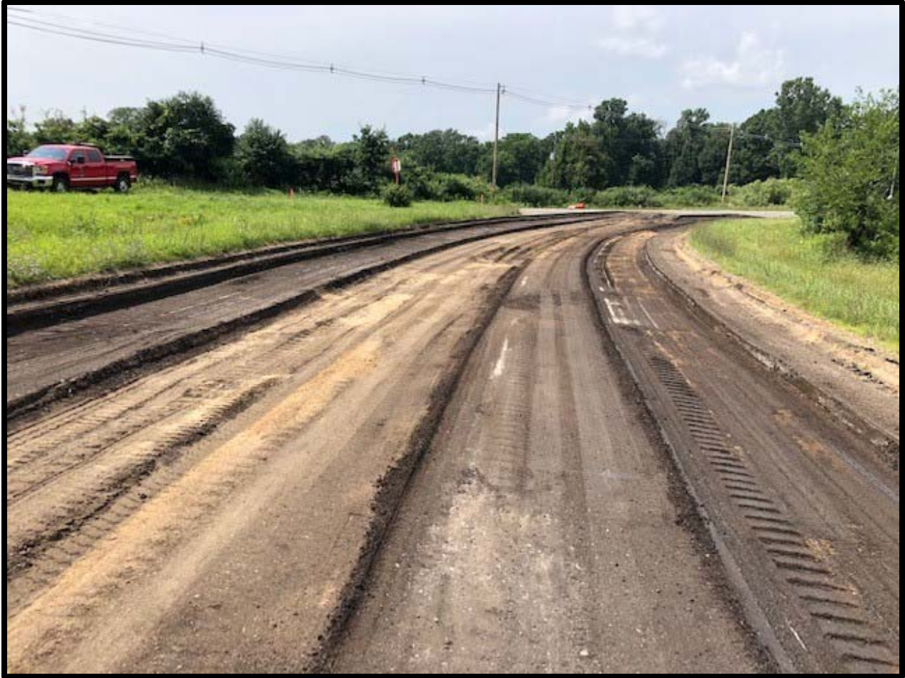
S. Jackson Road at Lindsey Road – Existing base after asphalt removal
