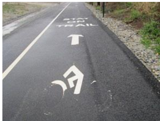
Pavement markings, Hanover Trolley Trail, PA.
