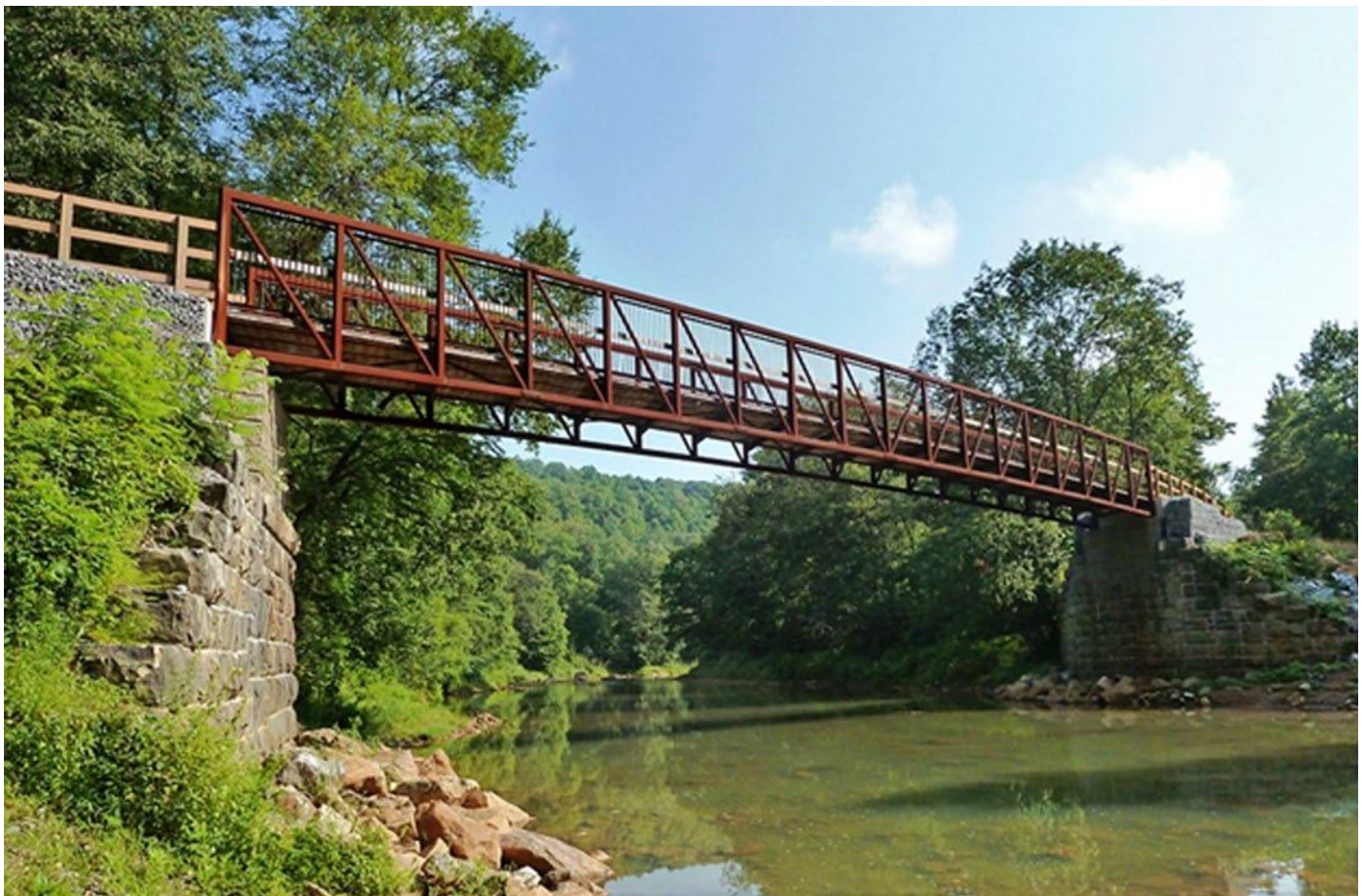
Scott Glen Bridge, Ghost Town Trail, PA.
