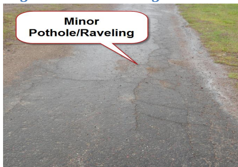
Figure Three: Raveling
