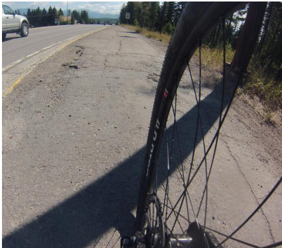
Figure Six: Shared Use Path-Poor Condition
