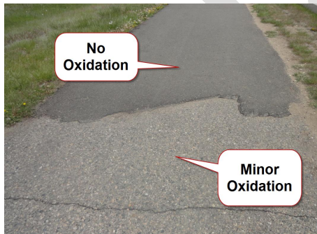
Figure Two: Oxidation
