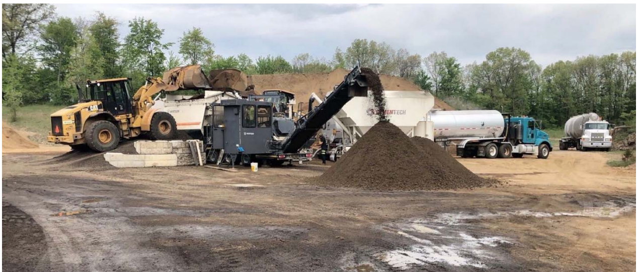
Cold central plant (KMA 220i) production at Blue Ridge Pit
