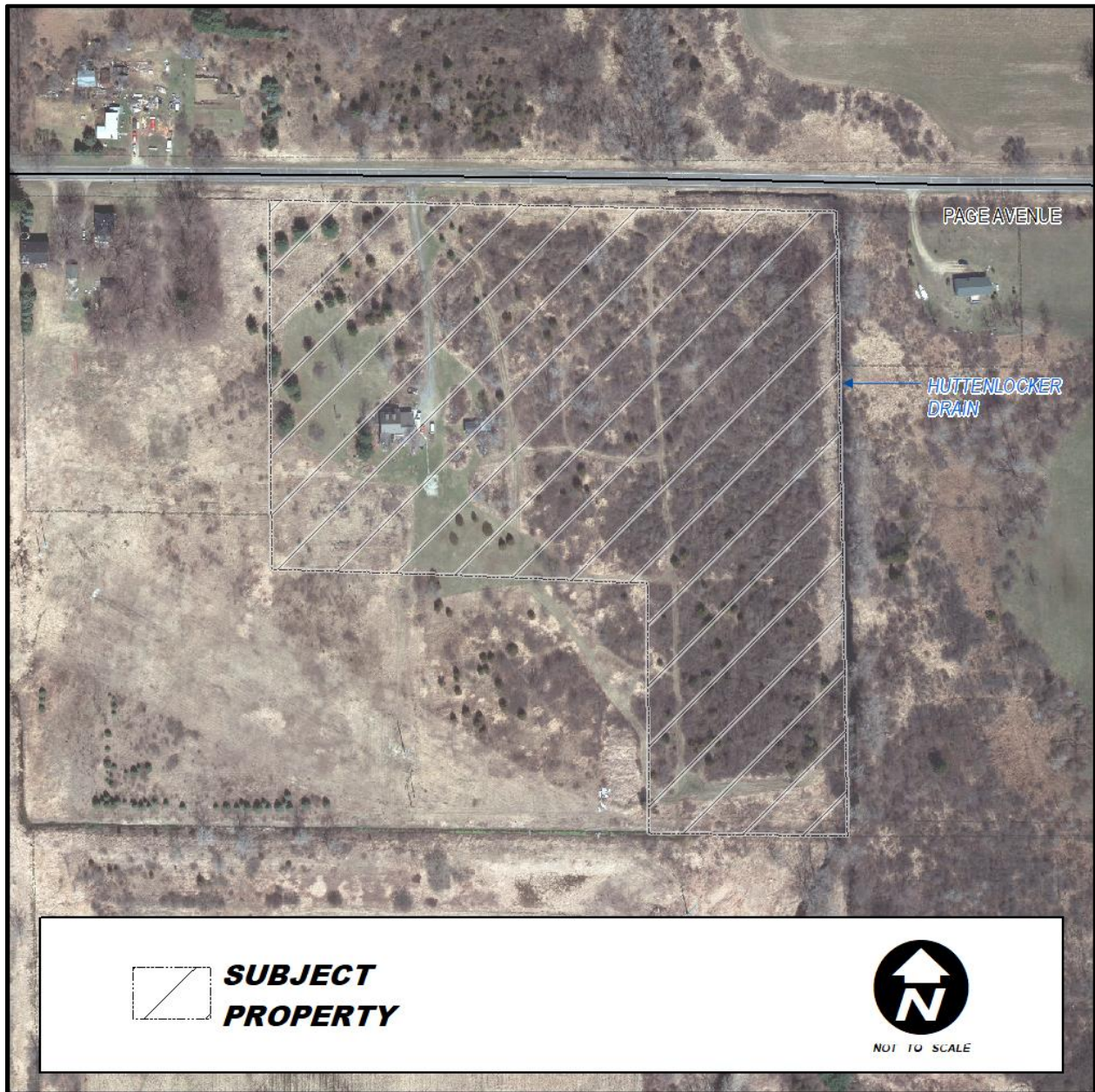
Figure 4b Aerial Photo
