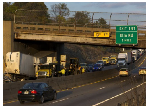
Figure 6-4 Cooper Street Bridge on I-94
