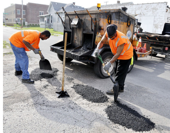
Figure 10-2 Filling Potholes
