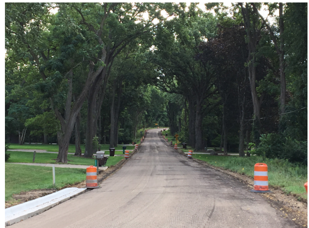
Robinson Road under construction
