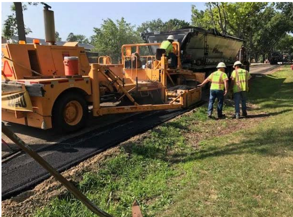
Paving the trenched areas on Robinson Road
