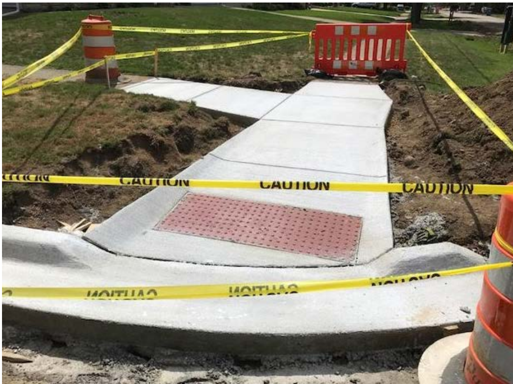
New ADA compliant sidewalk ramps on Robinson Road
