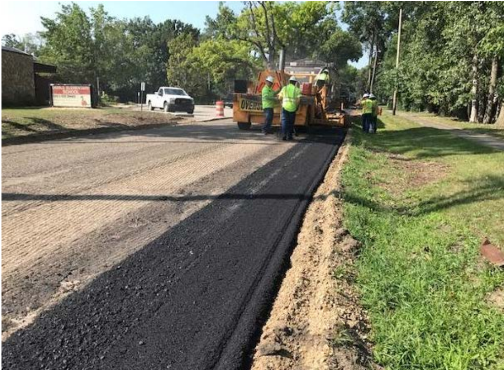
Paving the trenched areas on Robinson Road
