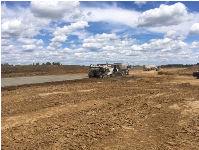
Treatment of wet sub base soils
